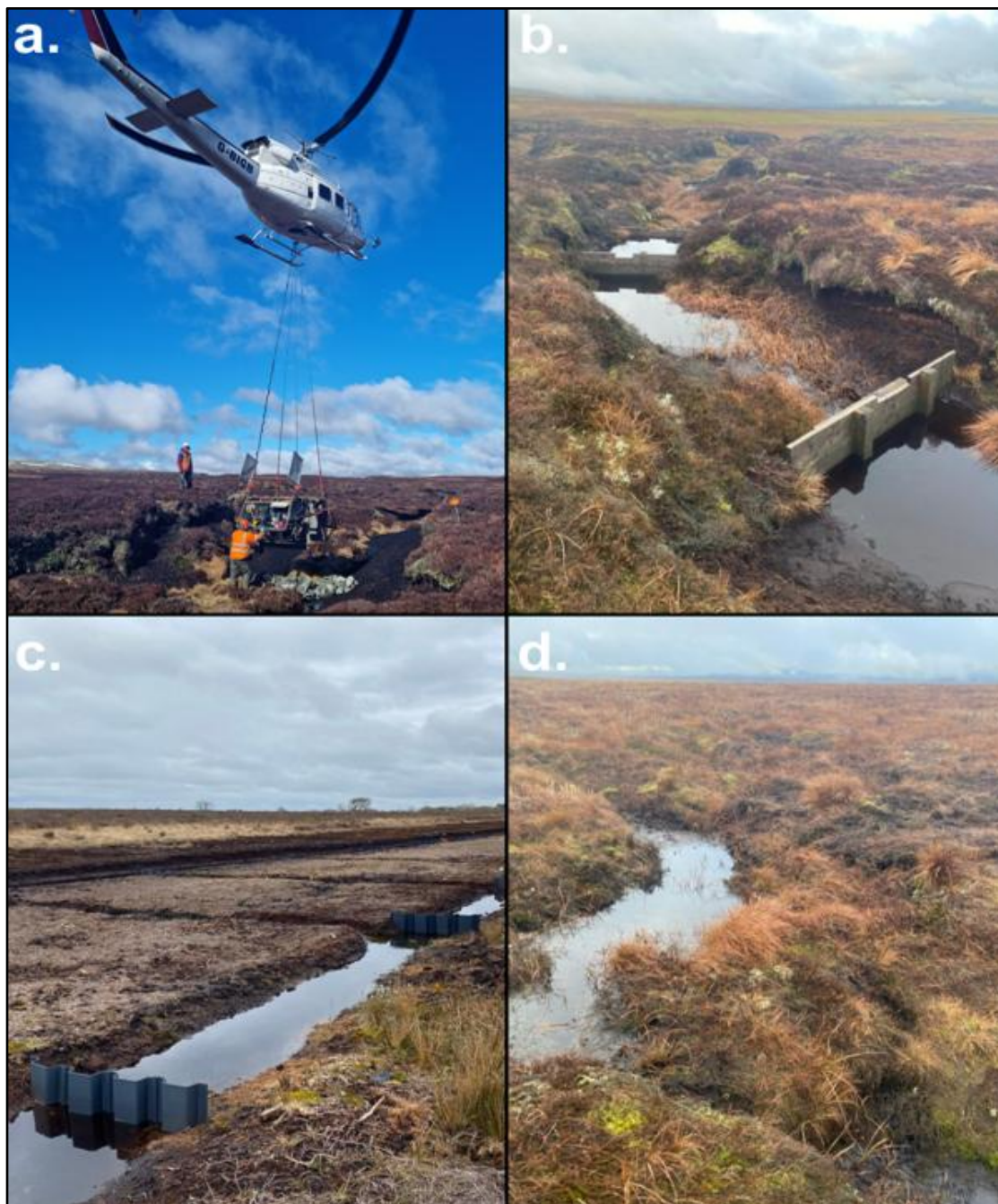
Figure 2.15: Examples of ditch and gully blocking interventions (Thom et al. , 2019; NatureScot, 2021): a. helicopter installation of a stone dam, used to block large erosion gullies; b. timber dam installed by hand, working as a water and sediment trap; c. plastic piling installed to block drainage ditches, inserted by hand; d. peat dam created using low-pressure ground machinery (excavator), supporting water retention and Sphagnum growth.
