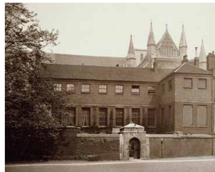
1 View of the exterior of Ashburnham House, 1880, by the photographer Henry Dixon (courtesy The British Library)
