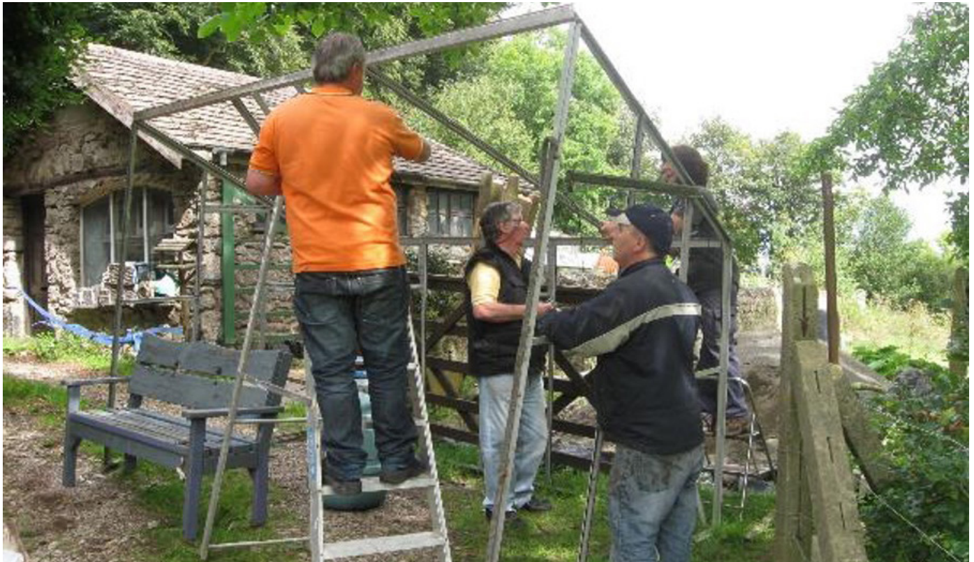
Figure 9. Constructing a greenhouse
