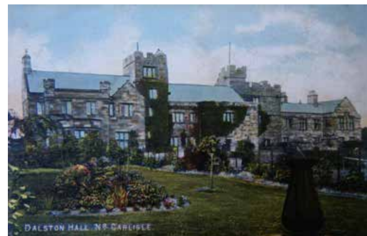
figure 2 – Dalston Hall c.1900 as remodelled by Carlisle architect C.J Ferguson for Edmund Wright Stead
