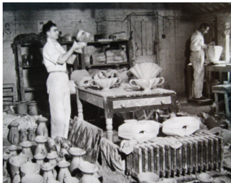
19. The drying room January 1952. Vases are left on the floor to harden prior to 'fettling'. No 'Constance Spry' shapes are to be seen and Marriner's FMA and FMC clearly outnumber the other vases present. Hammersmith & Fulham Archives and Local History Centre
