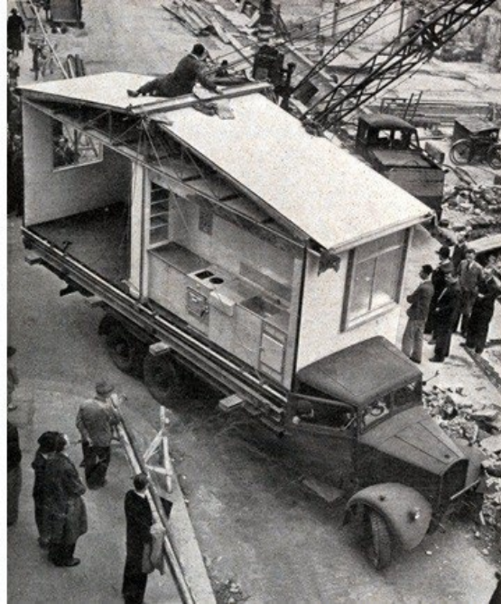
(Fig.3) A prefab arriving for assembly circa 1945
