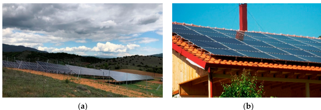
Figure 1. (a) Arnissa ground-mounted photovoltaic farm; (b) One of the five roof-mounted installations of 10 kW capacity.
