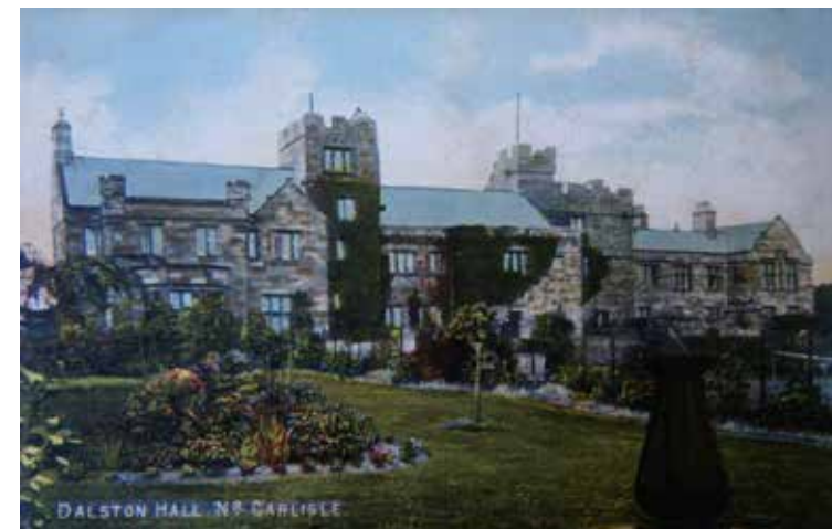
figure 2 – Dalston Hall c.1900 as remodelled by Carlisle architect C.J Ferguson for Edmund Wright Stead
