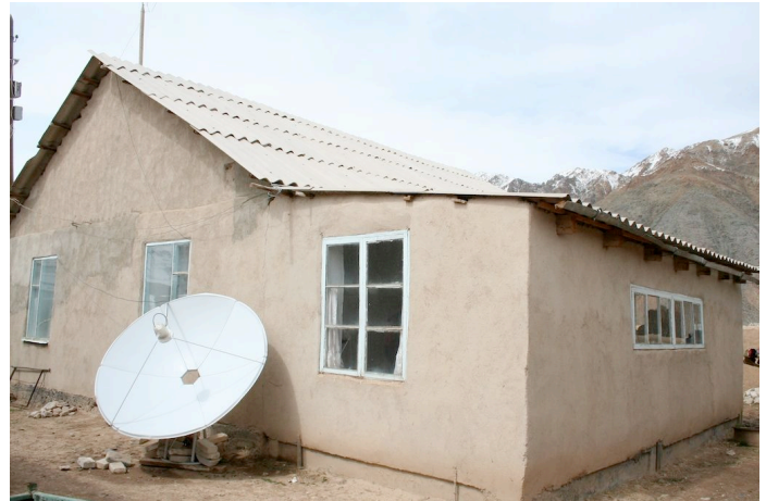
Figure 1 Satellite Dish, Tolok Village
