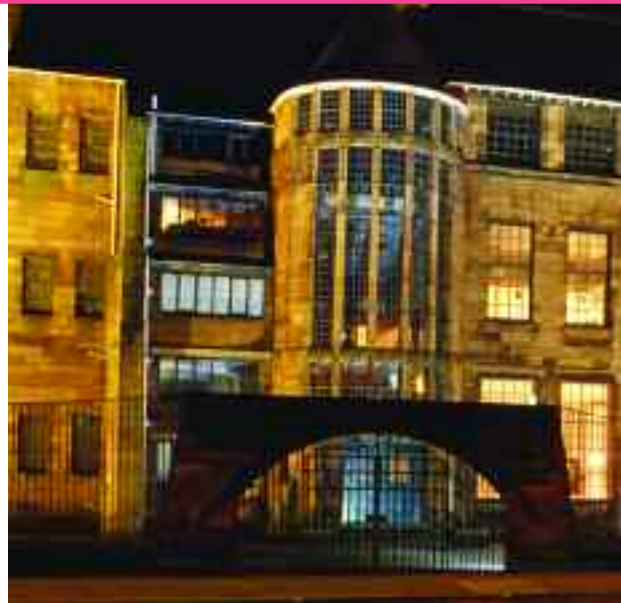
Scotland Street School at night
