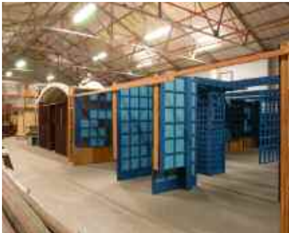
Restoration work in progress, 2002.
