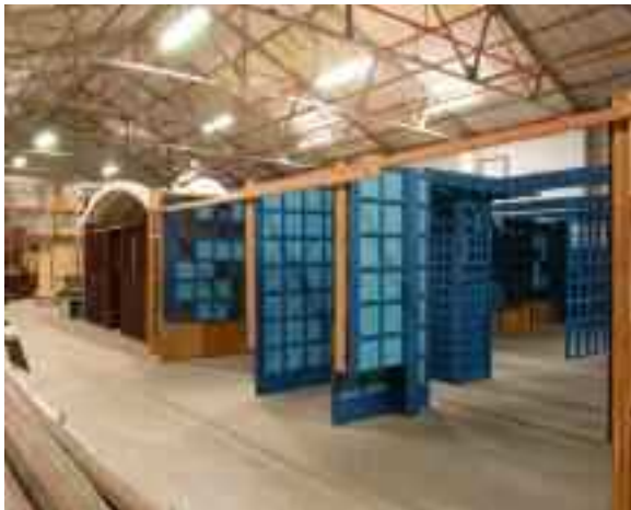
Restoration work in progress, 2002.
