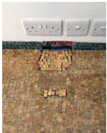
A trial section of new replacement tesserae laid dry.
