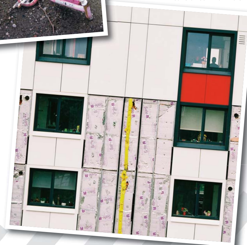
▶ Unsafe Tower Cladding, Salford – John van Aitken.
